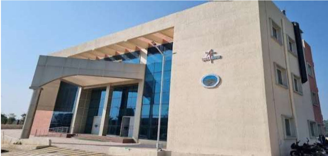
Department of ECE (ISRO Building), SDCSS Centre
