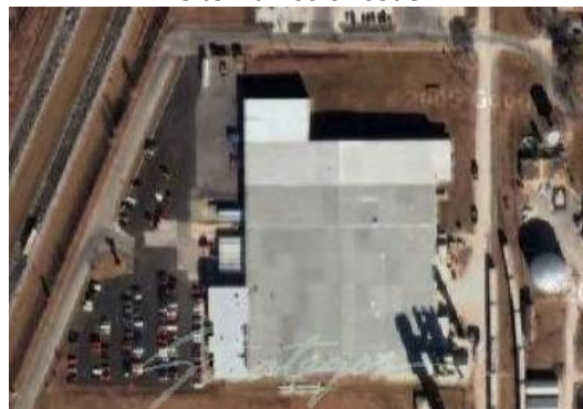
Satellite View of Vinyl-X Site
